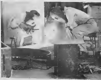
Welding operations require plenty of floor room. Lines run in gridded floor channels under new setup.
